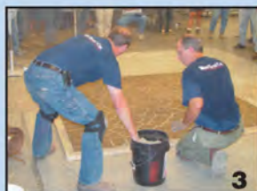
Add True Color™ Hardener and float concrete
