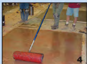
Add True Color Release™ and texture with roller
