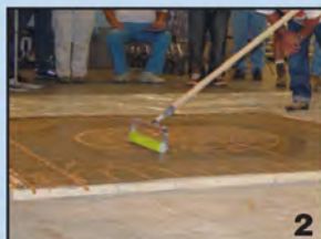
Embed stencil with roller
